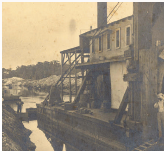
Dredging of the Everglades Source: Broward County Libraries Division Historical Archives
