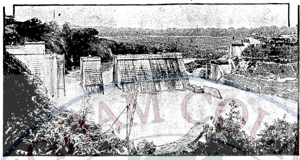
Flood waters of the Chagres river breaking through a section of the uncompleted Madden dam in Panama. Work this project is expected to be completed in 1934. Increased water storage for the Panama canal and better control of the wet season floods are two objects of building the dam.
