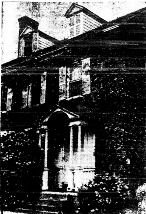
RECOGNIZED by architects as one of the finest examples of the Southern type porch in this area, the Smallwood-Ward "Town House" presents its features of art and culture to visitors of the annual New Bern pilgrimage.
