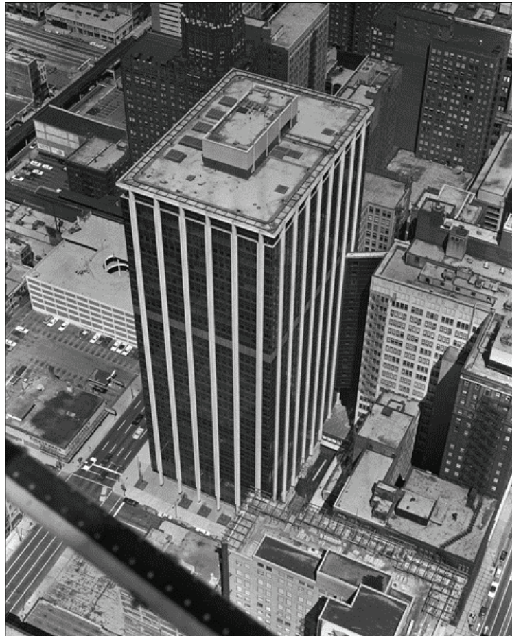
Aerial shot of the building circa 1970. The sky bridges on the south elevation at the sixth through 20th floors connecting it to the other Illinois Bell office building on W. Washington Street (located far right) are visible in this photo. (Source: Chicago History Museum)
