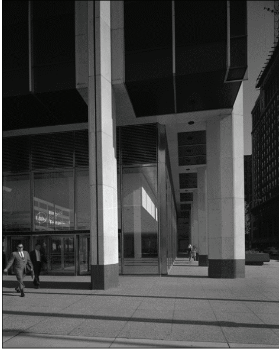
Photo of the northwest corner of the building circa 1966. The building's design features elements of the New Formalist style including the modern envisioning of the colonnade –like plaza at the street level and the use of rich materials like marble and granite on the exterior. (Source: Chicago History Museum)
