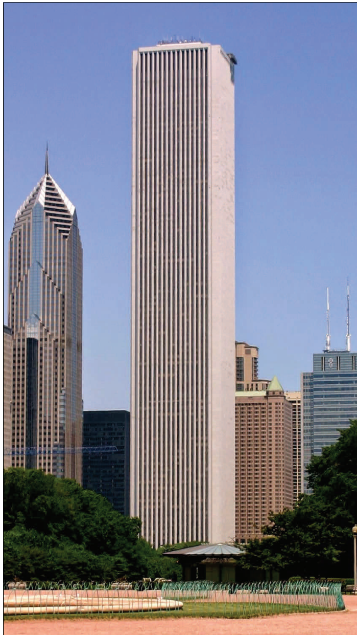
The 1974 Standard Oil Building at 200 E. Randolph Street was designed by Edward Durrell Stone and Perkins and Will. Originally clad in marble, the entire exterior cladding of the building was replaced with granite between 1990 and 1992. (Source: www.chicagoarchitecture.info )
