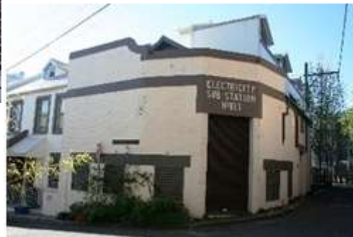
41. 1 Electricity Substation No 133, 32 Goodchap Street, Surry Hills, 1922 Source: http://www.environment.nsw.gov.au/heritageapp/ViewHeritagItemDetails.aspx?ID=3430401
