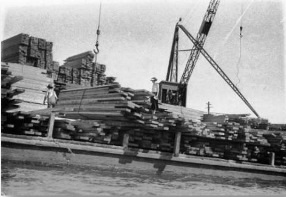
49. Stack of timber at Blackwattle Bay, 1930s Source: SLNSW hood_03584
