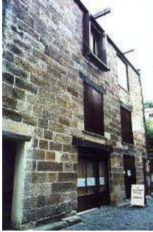
1. 1850s Warehouse, Kendall Lane, The Rocks Source: City of Sydney Archives 020\020758, Garry Deirmendjian, photographer.
