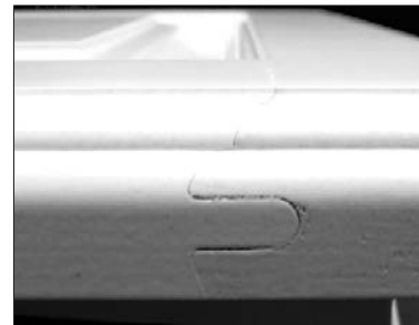
Example of end joint separation
