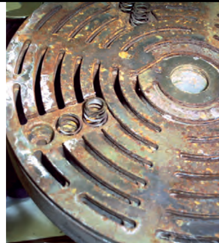
FIGURE 14 Corrosion in metal plate valve due to extended compressor shutdown period in a PET air compressor.
