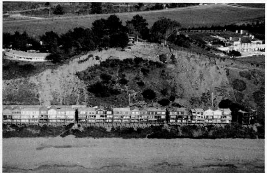
Photo 8. Very large dry sand flow above Place de Mer development. Houses at the top and base of this failure were at risk.
