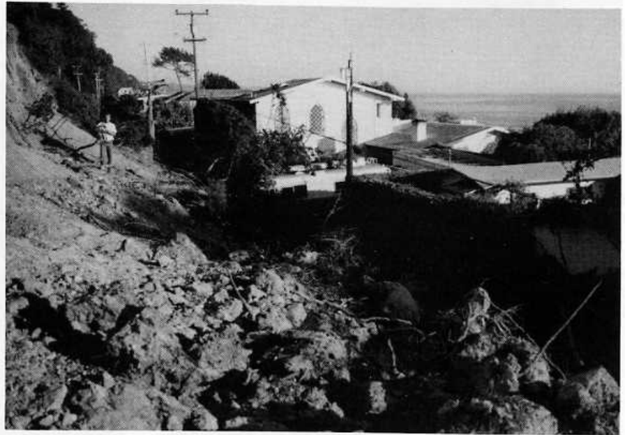
Photo 6. View facing east along Las Olas Drive. Material from a failure in the upper part of the bluff cascaded down the slope and blocked the road. Note the telephone pole broken by the landslide.
