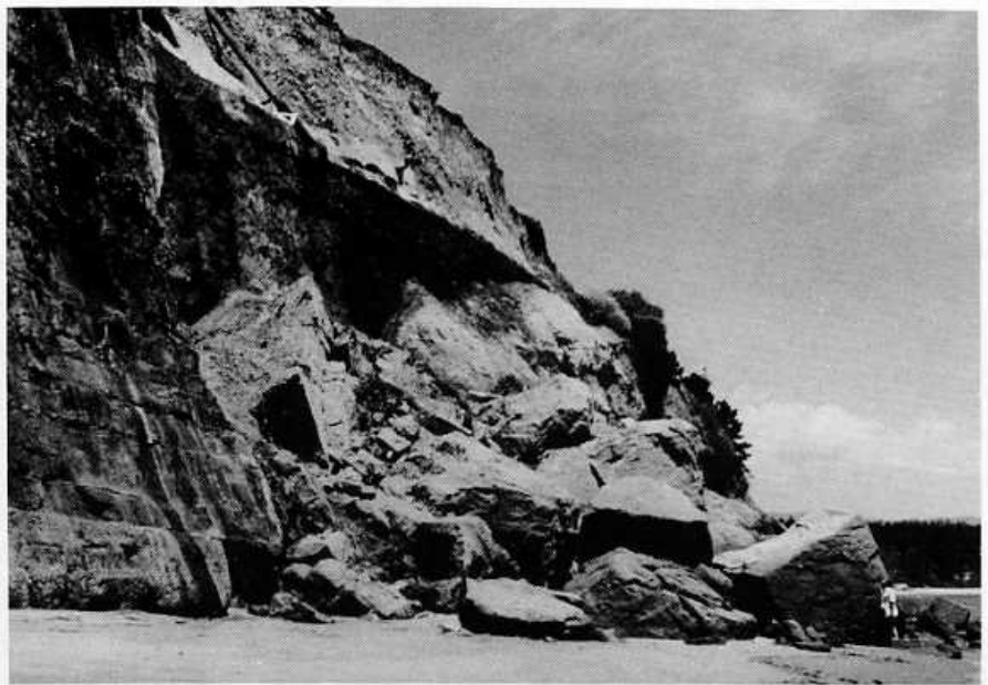
Photo 1. Joint controlled wedge failure in the Pliocene Purisima Formation. Marine erosion processes undercut these cliffs, which failed along intersecting joint planes.
