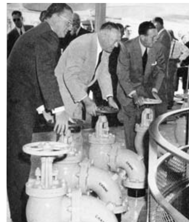
Below: A valve-turning ceremony opened the Crane “Tomorrowland” exhibit. From left to right: Henry Dreyfuss, designer of Crane plumbing fixtures and the exhibit’s “Bathroom of Tomorrow,” Frank F. Elliott, president of Crane Co., and Walt Disney.
