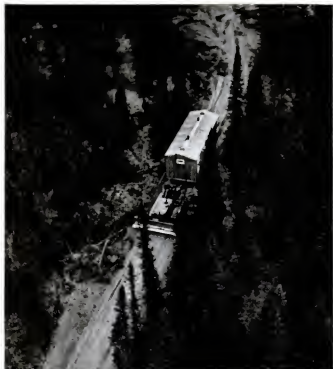
A CAT AND A COOKSHACK trundle up the road as soon as it is finished enough to hold them. After the cookshack, cabooses will be brought up for the men to live in until more road has been cleared ahead. Then they move up again.
