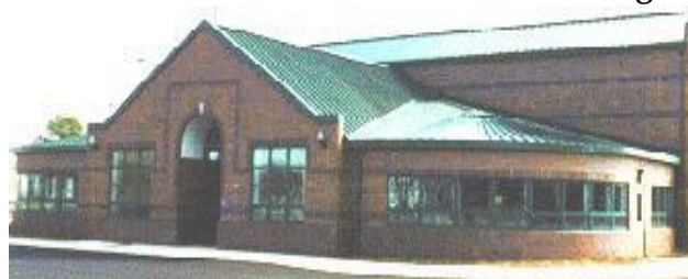
DPTS Administrative Office Building
