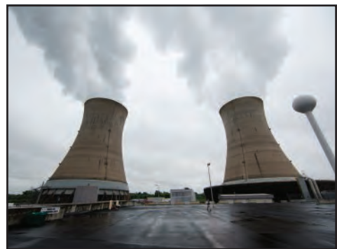
Cooling towers at the Three Mile Island nuclear power plant in Middletown, Pa.
