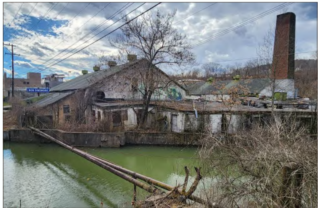
The Morgantown Utility Board purchased the former Dinsmore Tire property, at 195 Don Knotts Blvd., in early 2019 with the understanding the utility's neighboring water treatment facility would eventually need to expand. MUB is exploring use of the site as part of a water treatment plant project currently slated to begin in early 2025.
