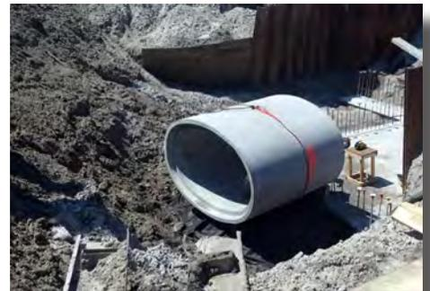
[Image 7-3] Drainage Pipe for Stormwater
