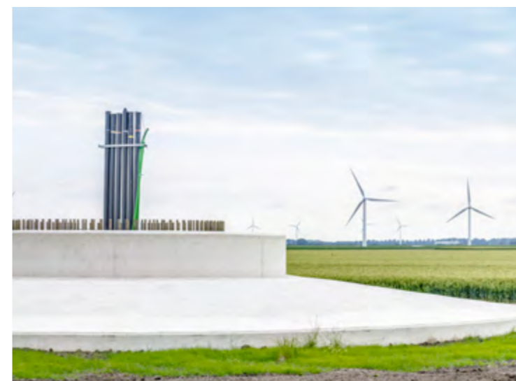
Foundation construction at Zeewolde
