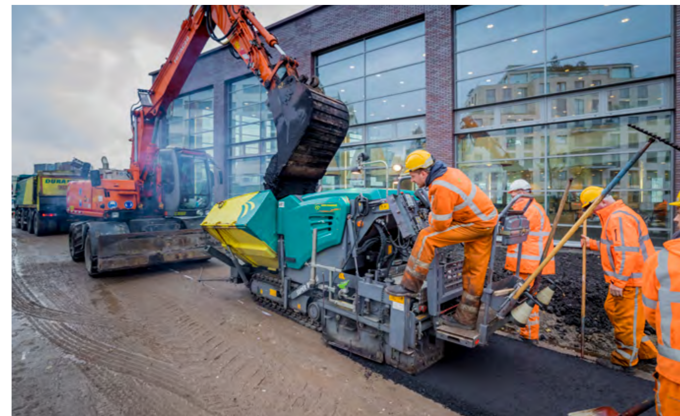
Asphalting work Overhoeks, Amsterdam
