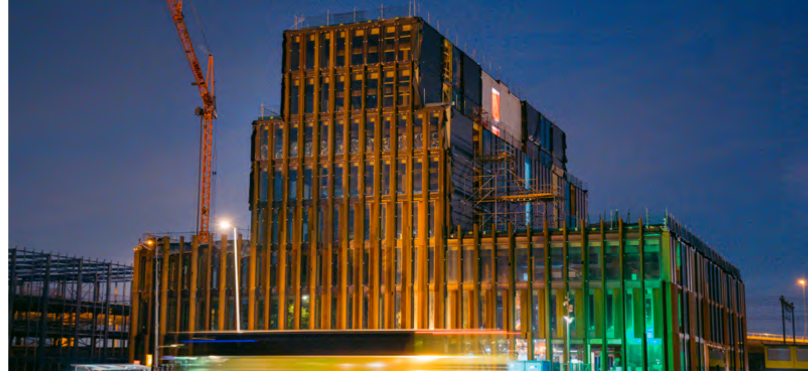
The timber-framed new regional office of Alliander, Amsterdam-Westpoort.
