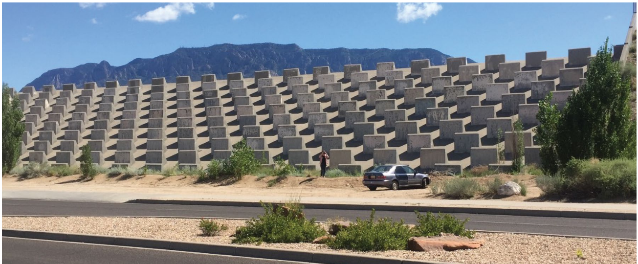
Figure 9.7. The emergency spillway for John Robert Dam, owned by the Albuquerque Metropolitan Arroyo Flood Control Authority. The spillway was designed to convey a flow of 23,600 cfs from a PMP storm. Photo by Bruce M. Thomson
