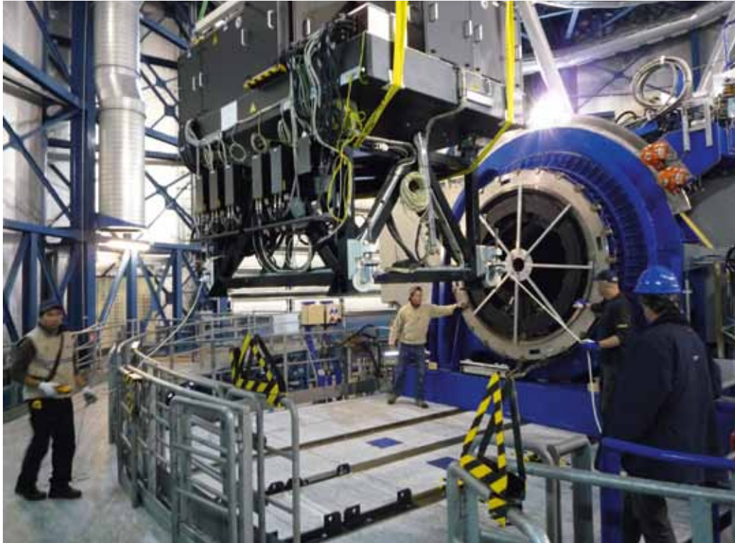
The APE instrument being lowered onto the Nasmyth platform of the 8-metre Melipal Unit Telescope, on Paranal.
