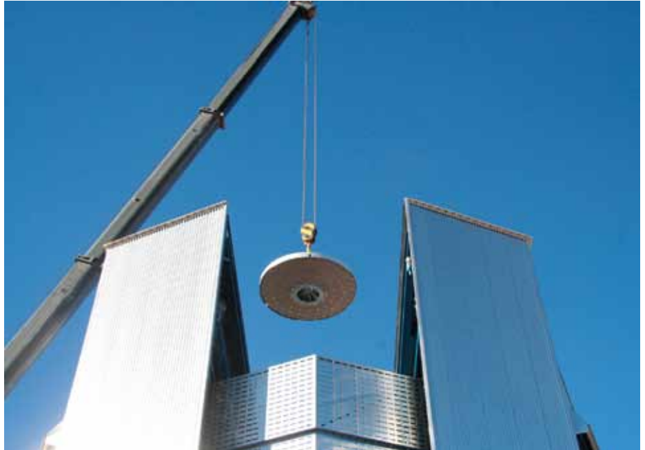
4.2-metre primary mirror being lowered into the VISTA telescope.
