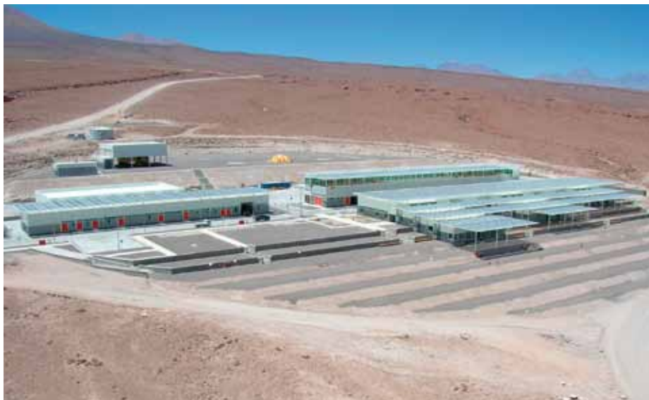
The Technical Facilities at the OSF.
