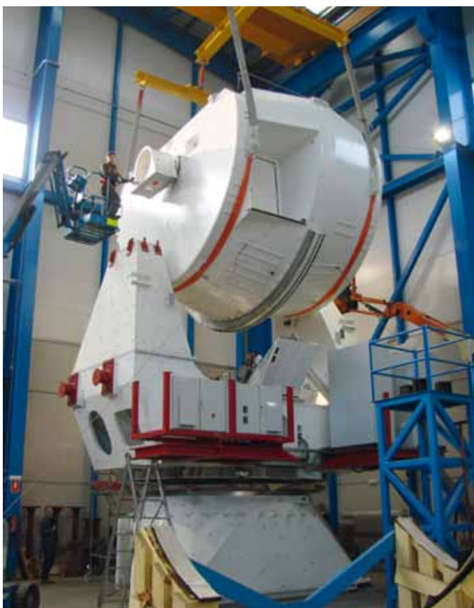
Assembly of the receiver cabin on the steel structure for testing in Europe.
