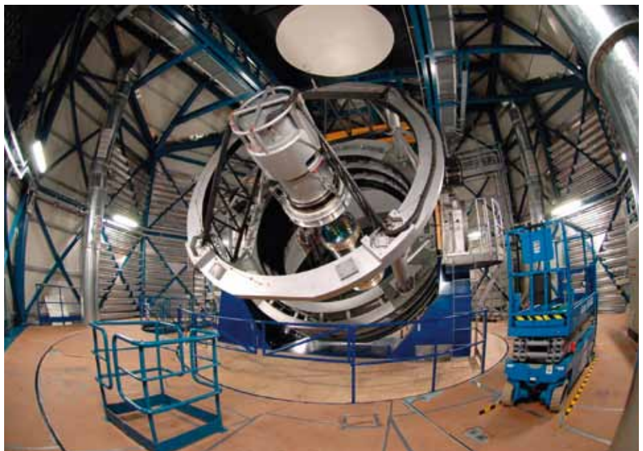
VISTA with all mirrors and camera installed.
