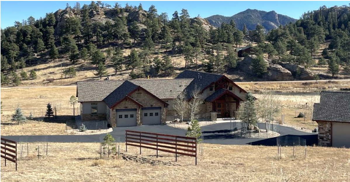
Top two photos: Tall grass and shrubs, tight crown space, and dense ladder fuels could endanger these upslope homes due to radiant and convective heating and short-range embers during a wildfire. Bottom two photos: Trees and shrubs near the homes are thinned, there is a 5-foot noncombustible zone around the structures, and the grass is mowed, making these homes more defensible and resistant to fire. Photos credits: The Ember Alliance.
