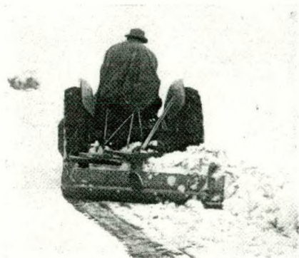
Ferguson Tractor and Earth Leveller keeping open a snow covered road.
