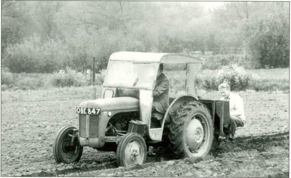
Most cabs restricted visibility, some more than others. The Scottish Aviation is one of the better types with a wide windscreen and the important small lower windows allowing a reasonable view of the front wheels. Robin Barker
