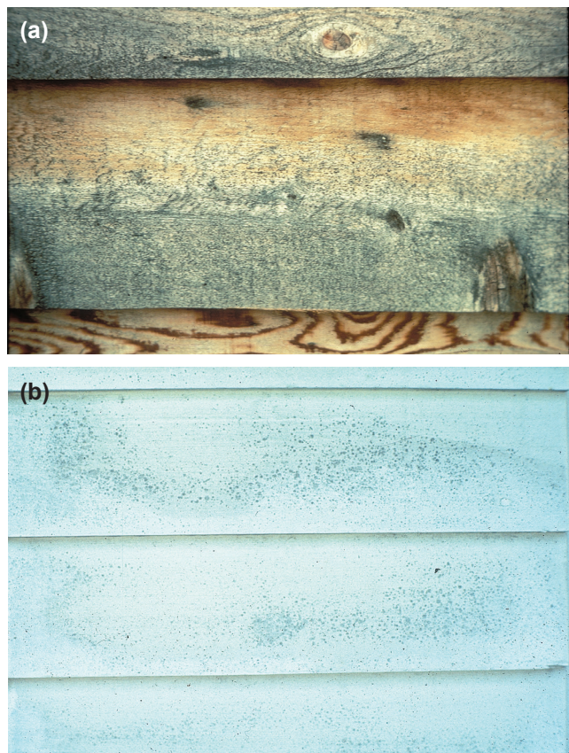
Figure 16–28. Mildew is most common in shaded, moist, or protected areas (a) on wood and (b) on painted wood.
