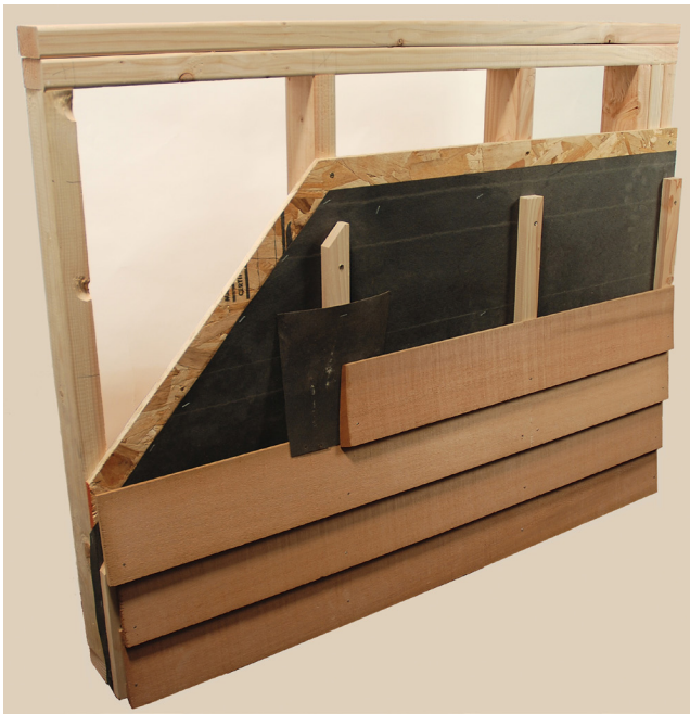
Figure 16–17. Demonstration of siding installation over a secondary drainage plane (rain screen) showing wall studs, sheathing, water-resistive barrier (WRB), and furring strips. Note that the butt joint is centered directly over the furring strip, a piece of water repellent barrier (felt) is added to drain water to the outside, and the end grain has been sealed.
