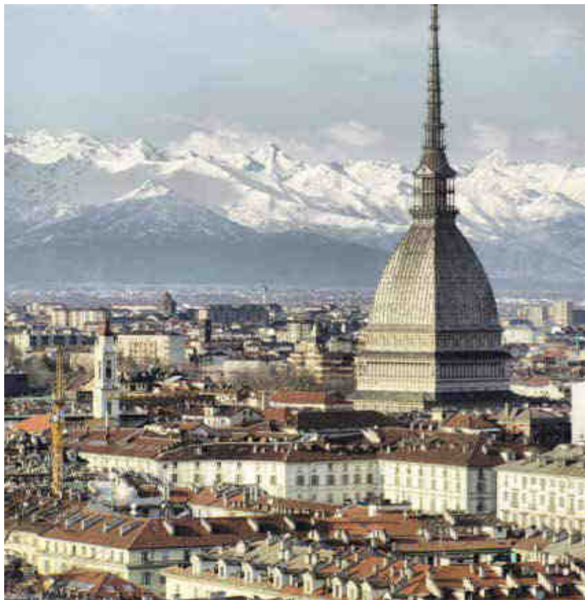
External facades - West elevation on Reale Mutua, Corso Siccardi - Turin (ITALY)
