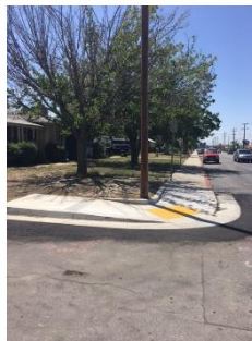
Curb cut constructed at Bernard/Magnolia Bus Stop
