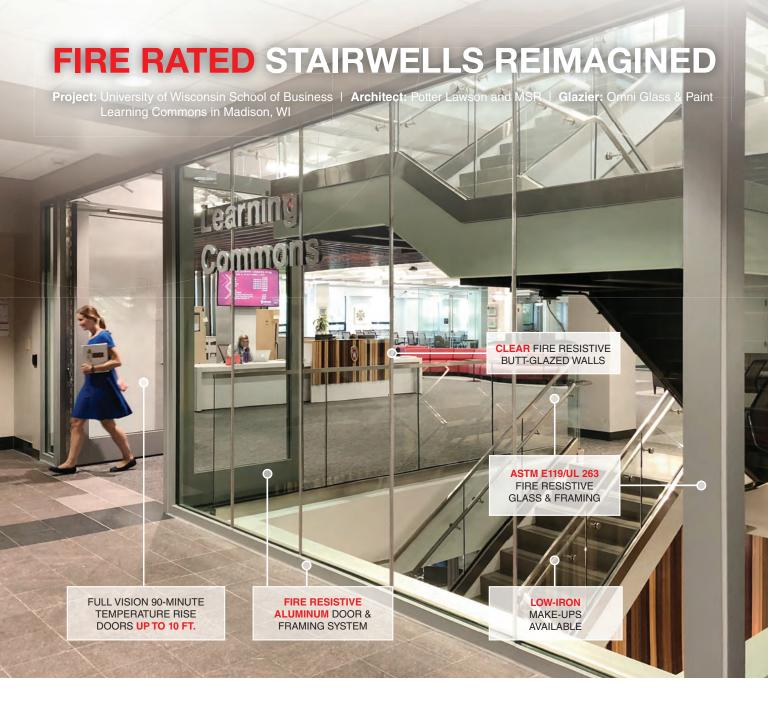
This stairwell maximizes daylight and transparency without compromising fire safety with **SuperLite**<sup>®</sup> **II-XLM 120** clear butt-glazed walls in **GPX**<sup>®</sup> **Architectural Series** perimeter framing. **SuperLite**<sup>®</sup> **II-XL 90** in **GPX**<sup>®</sup> **Architectural Series Aluminum Doors** provide a sleek, full-vision entrance system that compliment the overall aesthetic.
