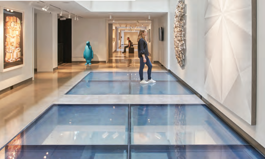
60-minute fire-resistive glass floor, the GPX FireFloor System by Safti First, at the 21c Museum Hotel in Nashville. Photo by Mike Schwartz Photography.
