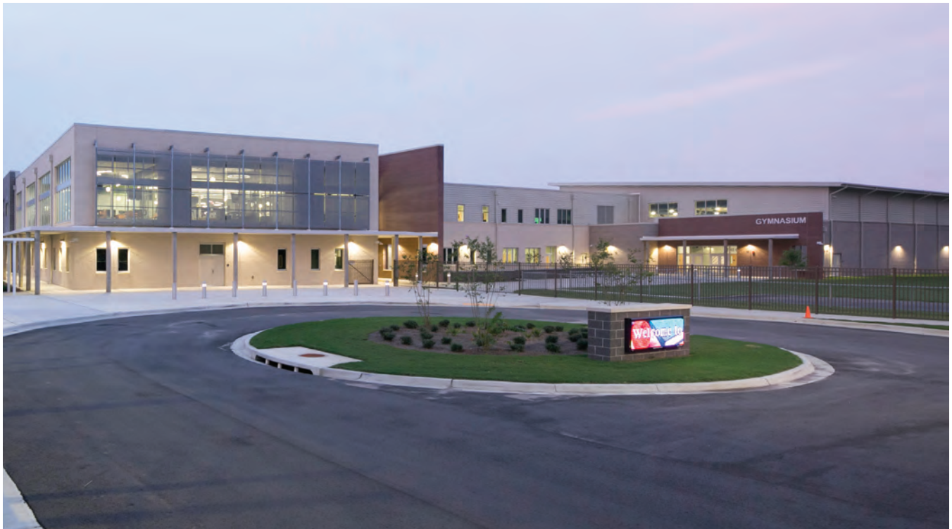
Protective laminated glass is featured on a middle school in Florida. The project features Saflex Acoustic PVB interlayer and Saflex Storm PVB interlayer from Eastman. The glass fabricator was Viracon. The architect was DAG Architects. Photo by Shawn Sandusky.
