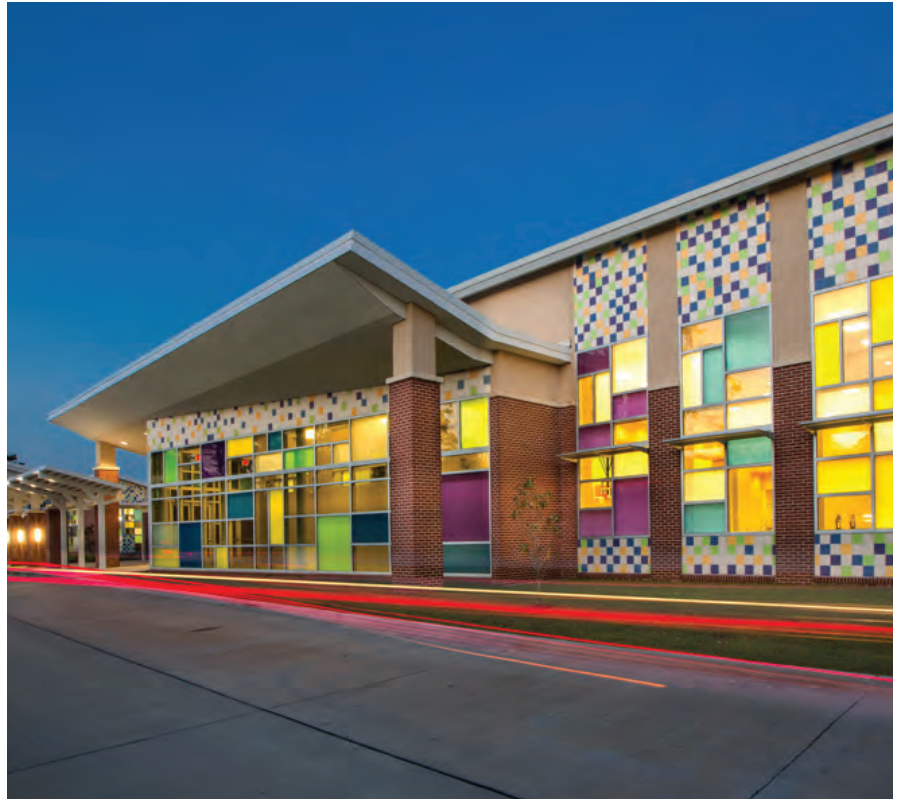
An elementary school in Louisiana. The school features safety glass from Viracon, laminated with Vanceva Colors PVB interlayer from Eastman Chemical Co. The architect was Coleman Partners Architects. Photo by Miami in Focus Inc.
