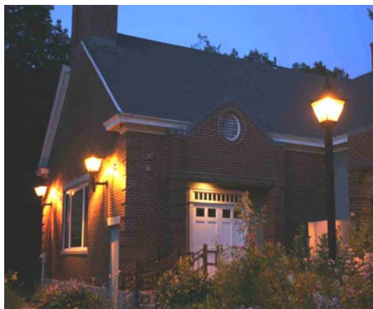
Library facade – fully shielded fixtures provide good illumination where it is needed – on the ground
