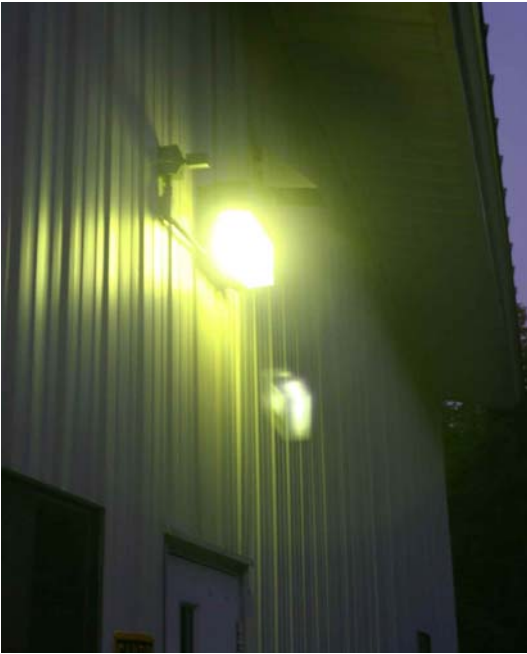
Poorly shielded “wall-pack” light causes dazzling glare at a local fire station
