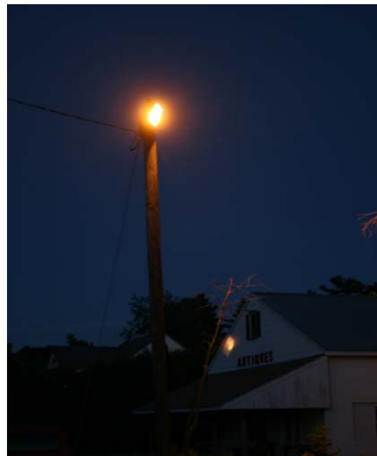
Angled, poorly shielded floodlight causes upward and down-street glare
