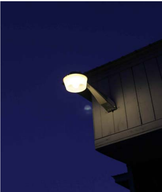
Popular mercury vapor/metal halide light fixture causes intense glare and sky pollution
