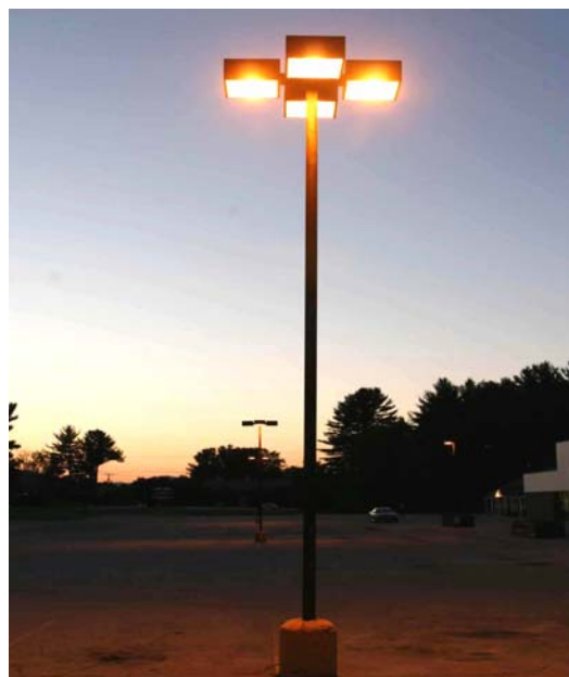
Shopping mall parking area - fully shielded provides good lighting without glare or sky pollution
