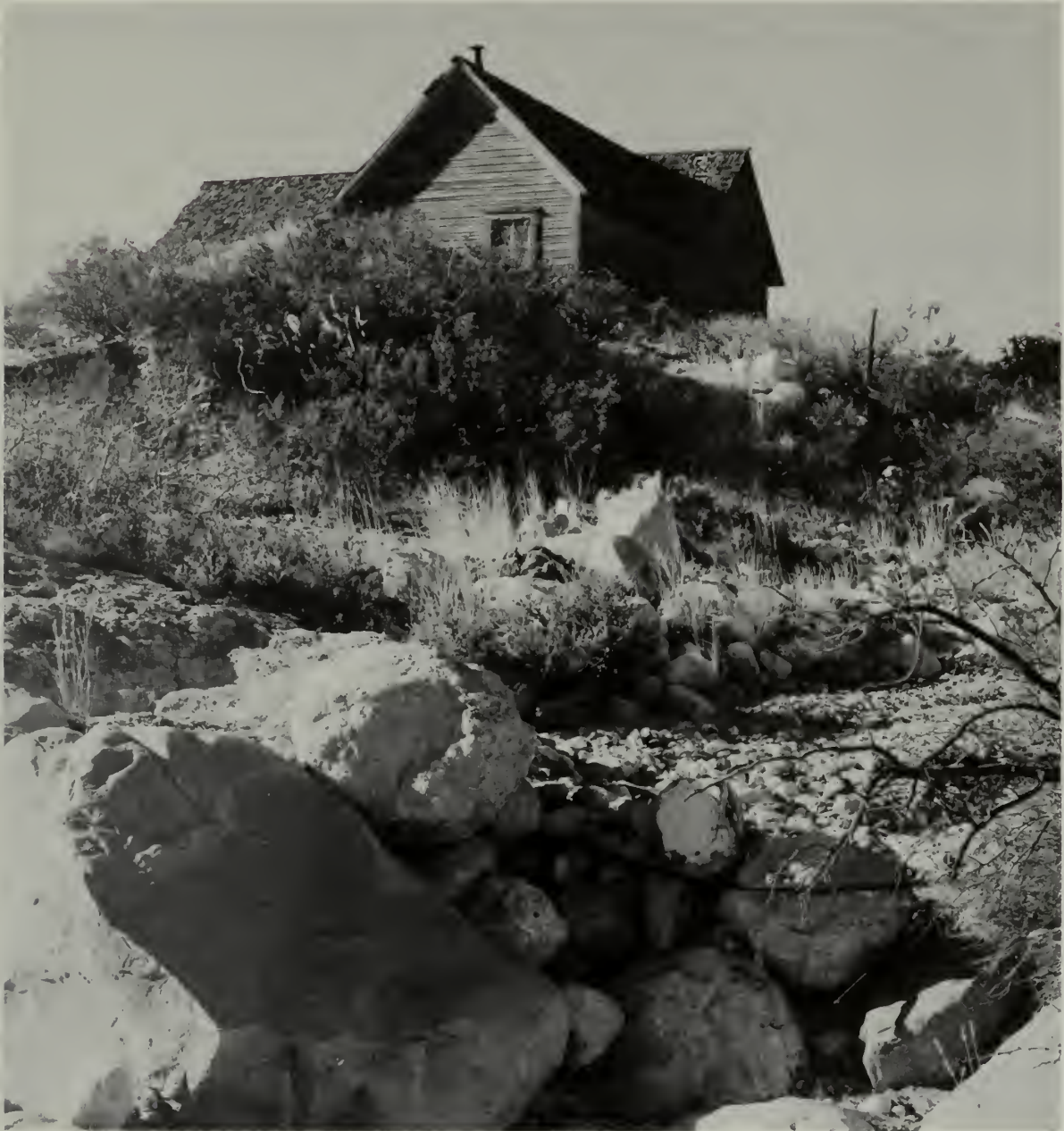
Figure 34. Another view of the Williams ranch house. Its architectural design makes it an anomaly on the West Texas landscape. (NPS Photo)
