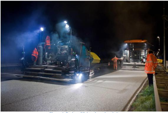
Figure 4: Paving of light coloured asphalt
