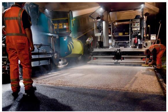
Figure 2: The first metres with clear binder (section C) on A35
