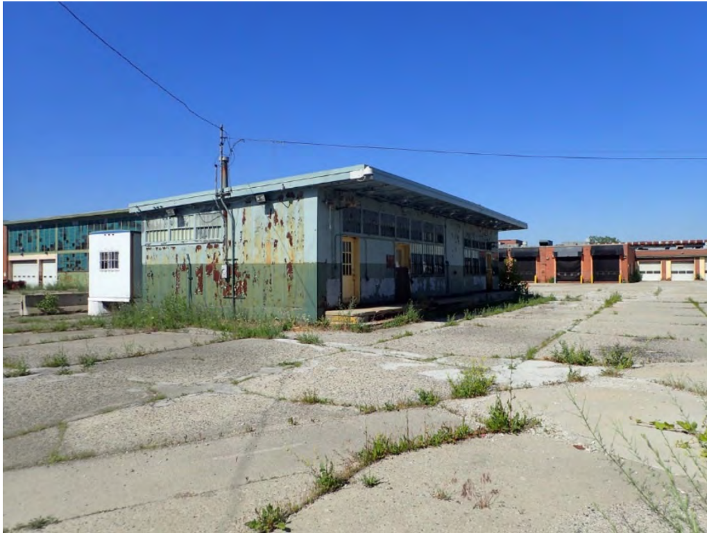
Photo 21. 14044 Schaefer Highway, Coolidge Fare Box House
