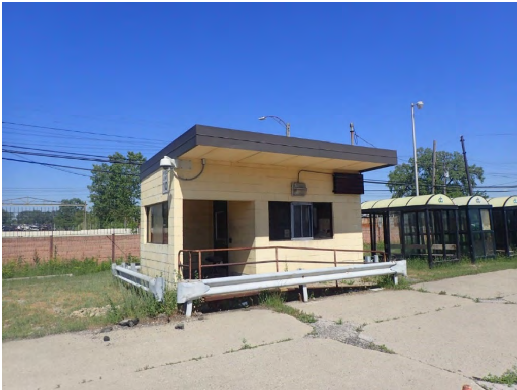
Photo 22. 14044 Schaefer Highway, Dispatch Building
