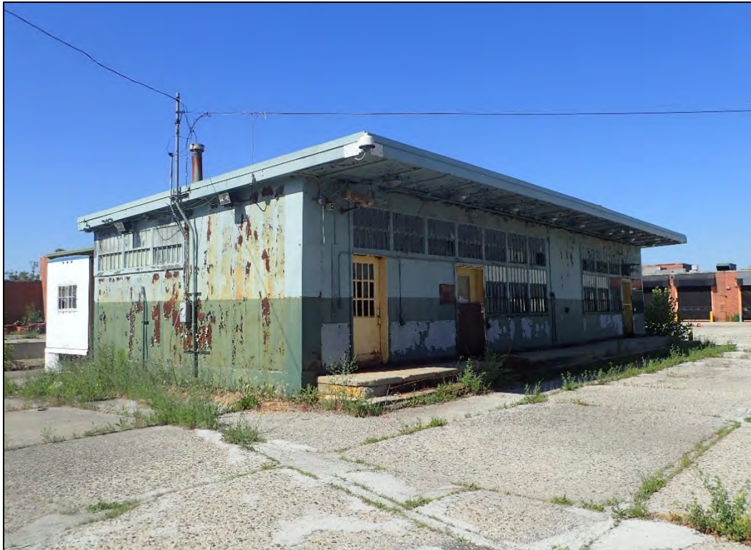
Figure 18. Fare Box House, view looking southwest.
