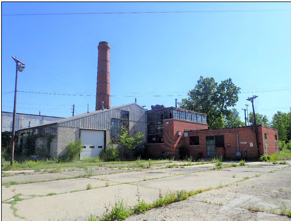
Figure 17. Heating plant, view looking northeast.
