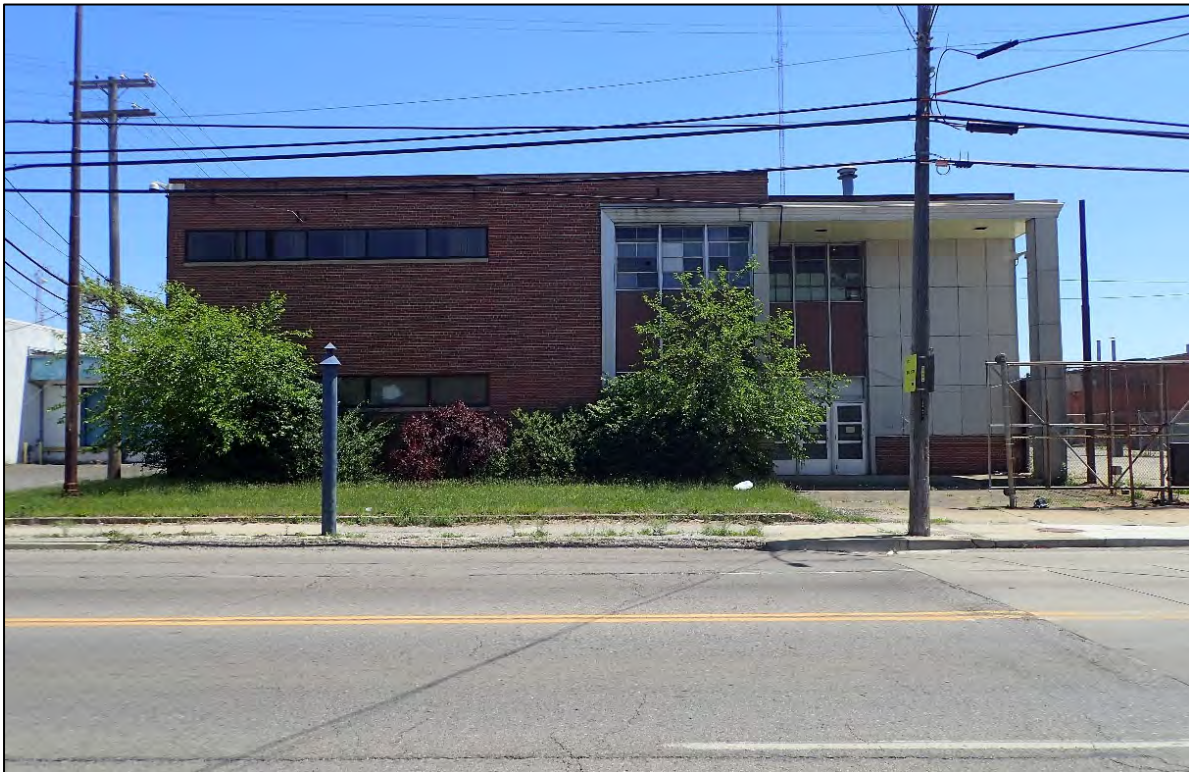
Figure 15. Building façade, view looking east.
