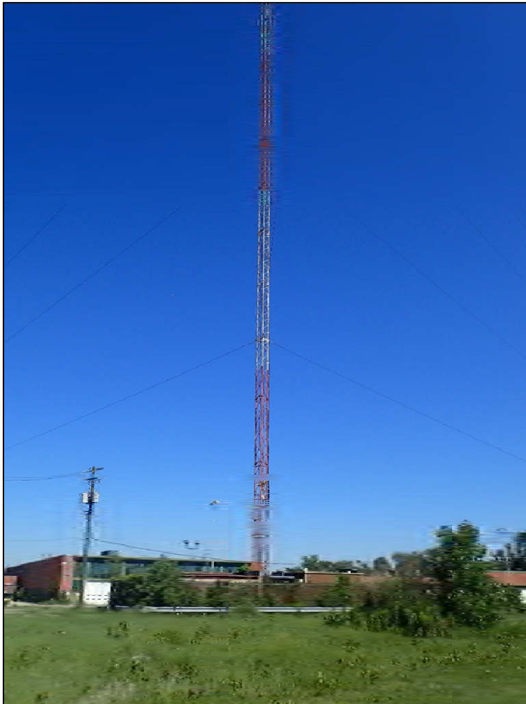
Figure 20. Communications facility, view looking southwest.
