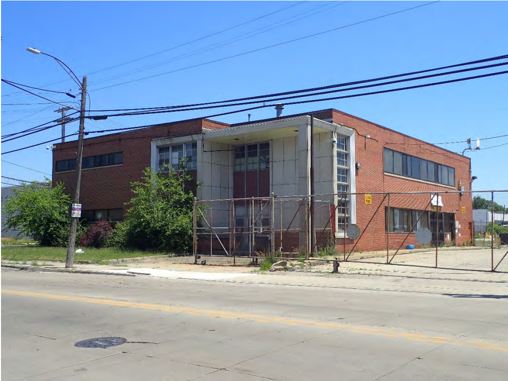
Photo 18. 14044 Schaefer Highway, Coolidge Administrative Building
