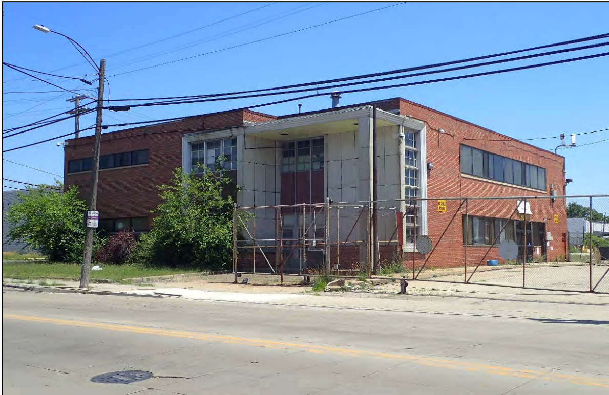
Figure 14. Coolidge Administrative Building, view looking northeast.
