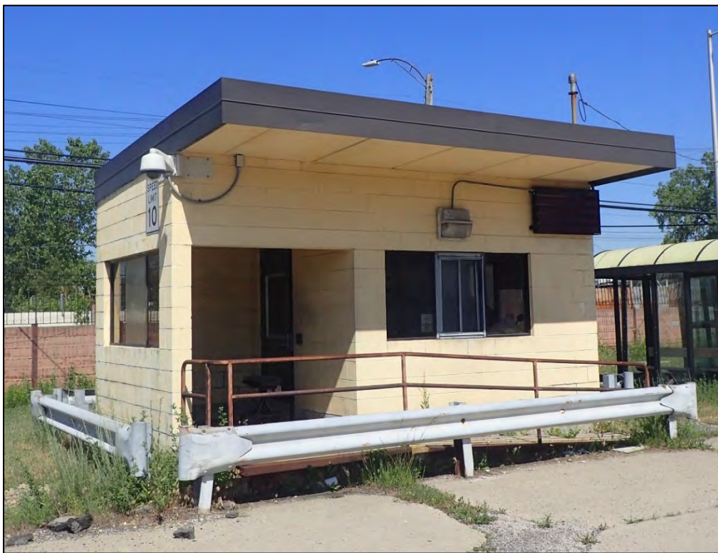
Figure 19. Dispatch House, view looking northwest.
