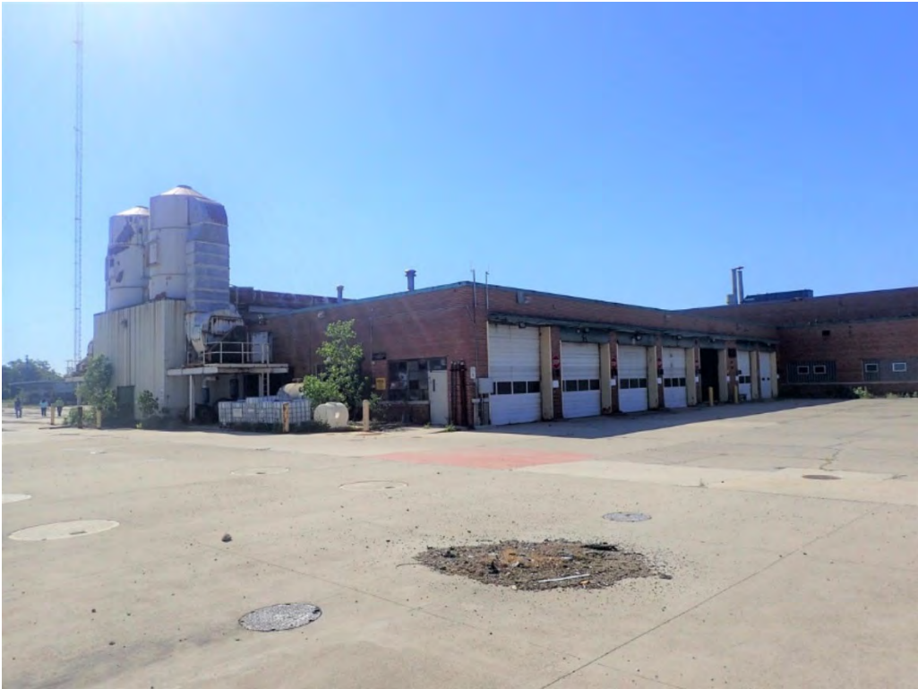
Photo 17. 14044 Schaefer Highway, Coolidge Terminal Building
