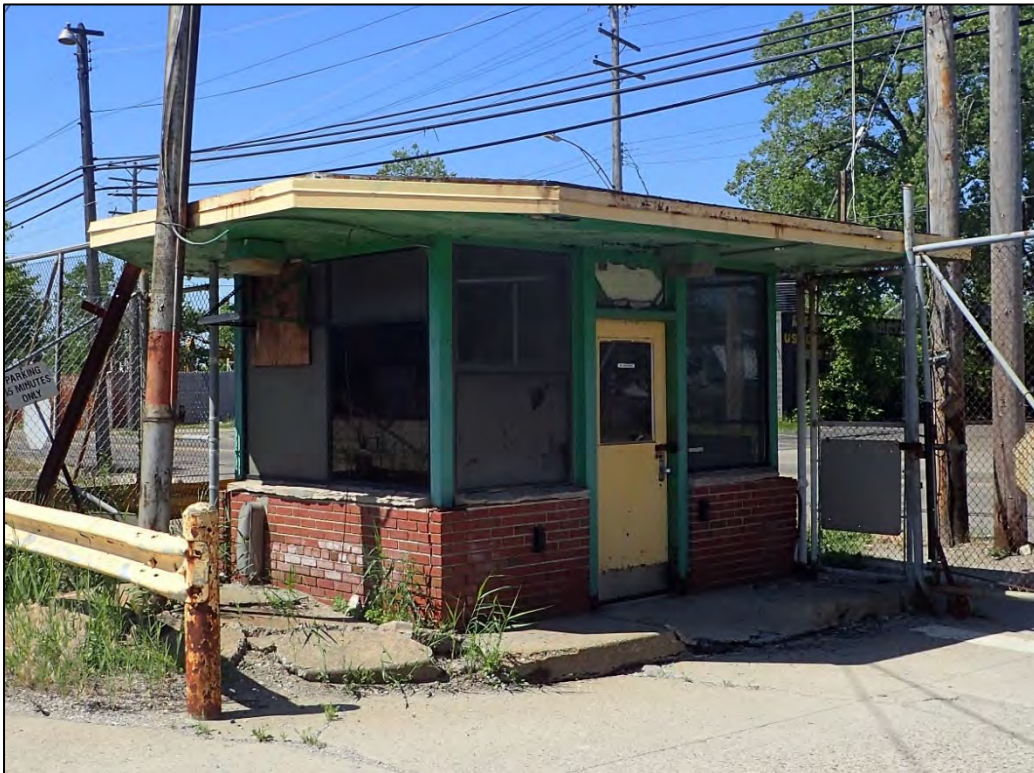
Figure 16. Gatehouse, view looking southwest.
