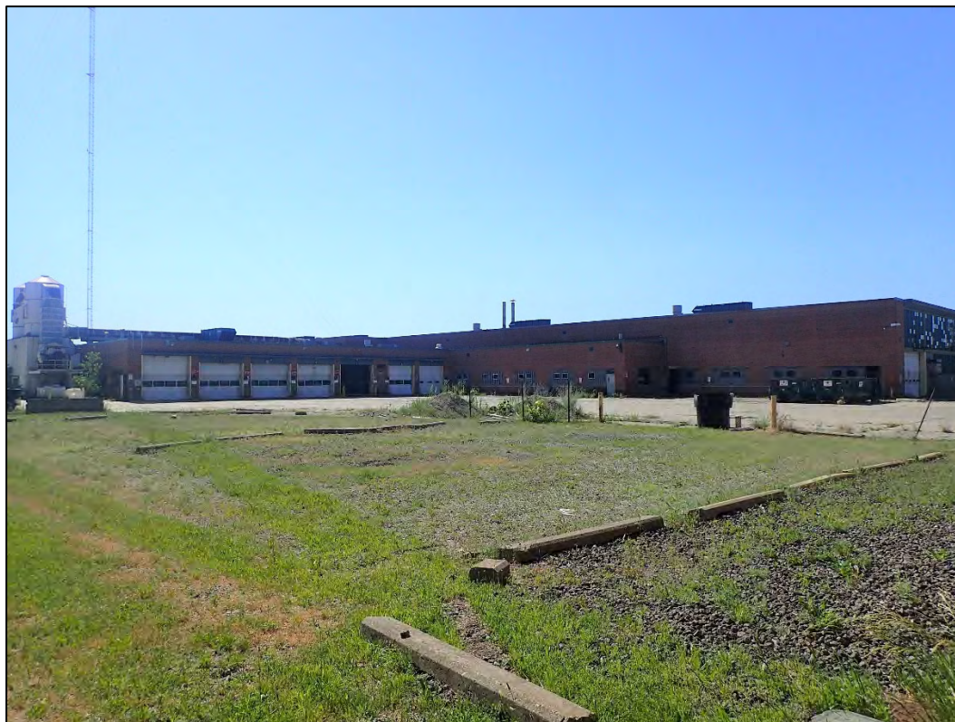
Figure 13. View looking southeast. Visible at left is the washing wing; at right is the bus garage.
