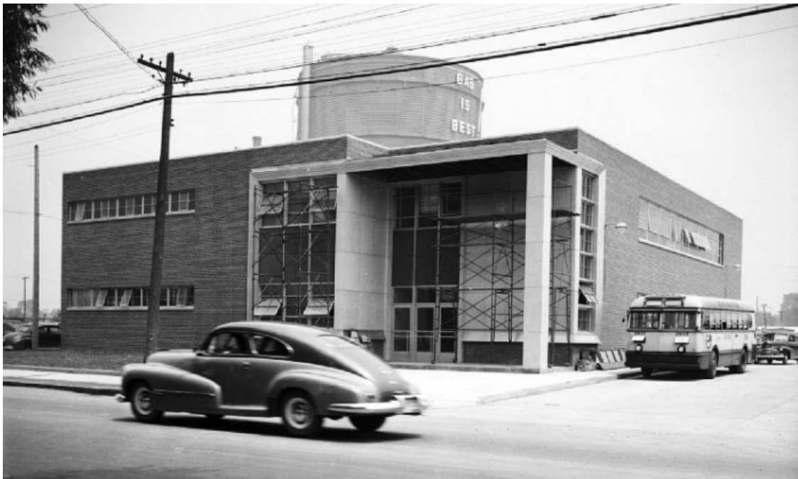
Figure 7. Coolidge Terminal Administrative Building, June 22, 1948 (Craig 2010).
