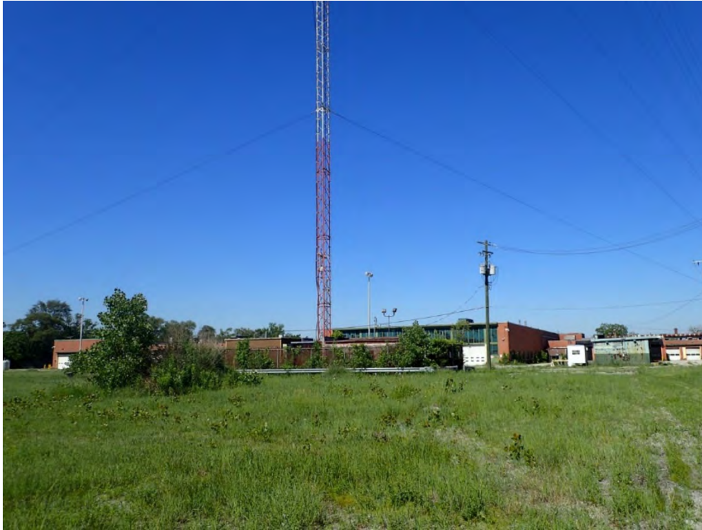
Photo 23. 14044 Schaefer Highway, Communications Facility
