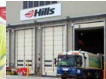
The Northacre Resource Recovery Centre in Westbury.
