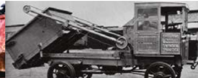
An early brick delivery lorry. This four-wheel drive vehicle had a mechanised container for tipping its entire load.
