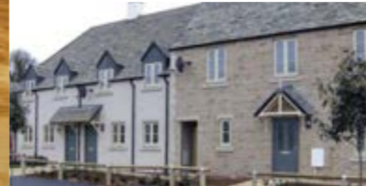
Traditional building skills and the most up to date green technology create sustainable and efficient modern homes.
