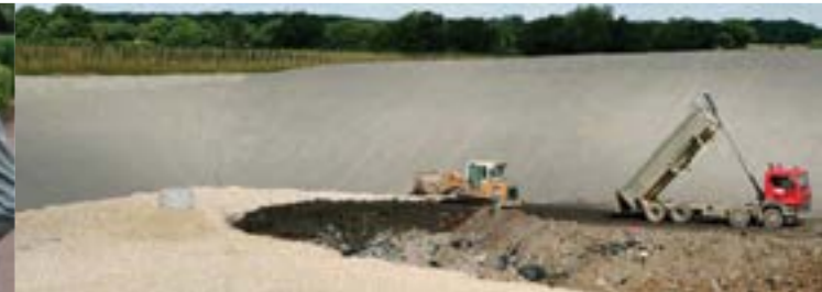
A landfill site is constructed to stringent Environment Agency standards.
