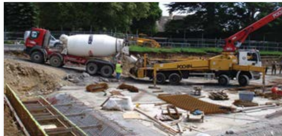
Quarry Products' ready-mixed concrete is pumped on to a construction site.
