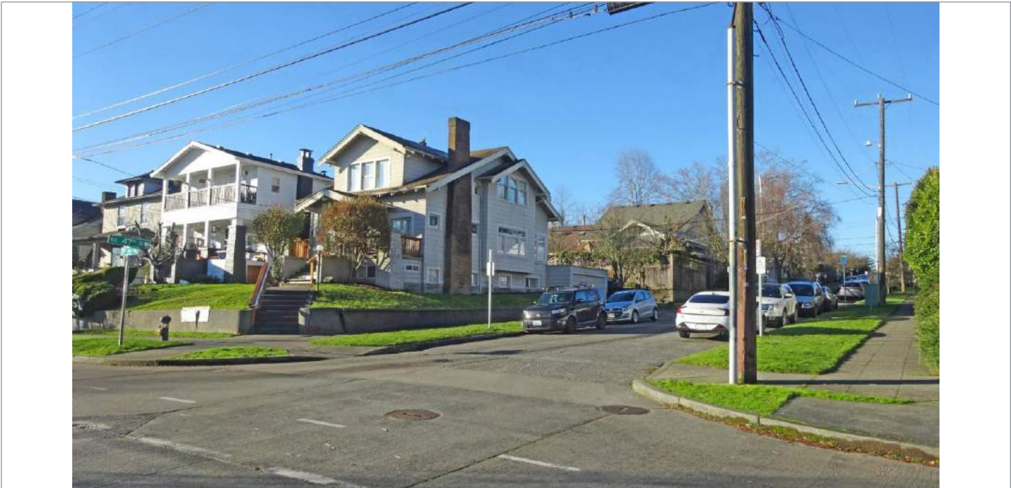
WA_King County_Wallingford-Meridian_Streetcar_HD_0055. NE, looking southwest.
