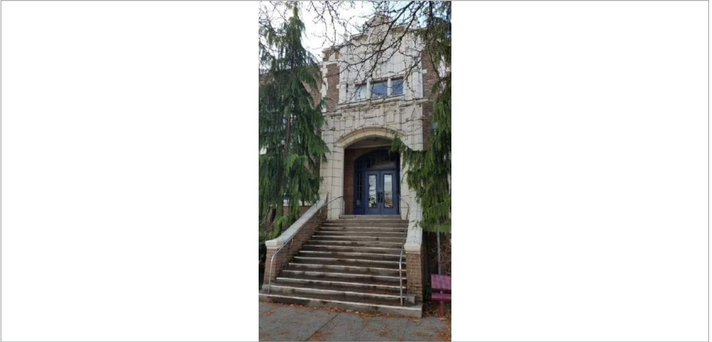
WA_King County_Wallingford-Meridian_Streetcar_HD_0011. west.
