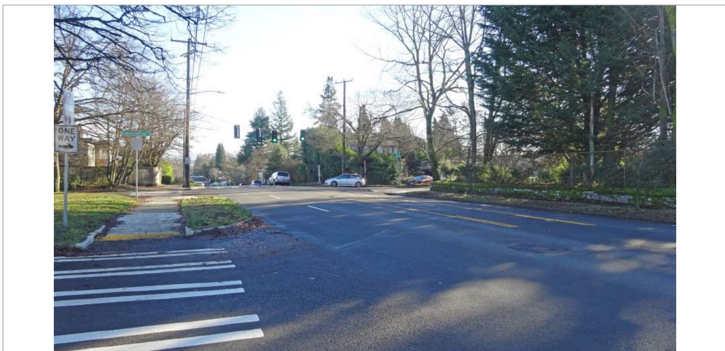
WA_King County_Wallingford-Meridian_Streetcar_HD_0032. Intersection of N 50th Street and Sunnyside Avenue N, looking southeast.
