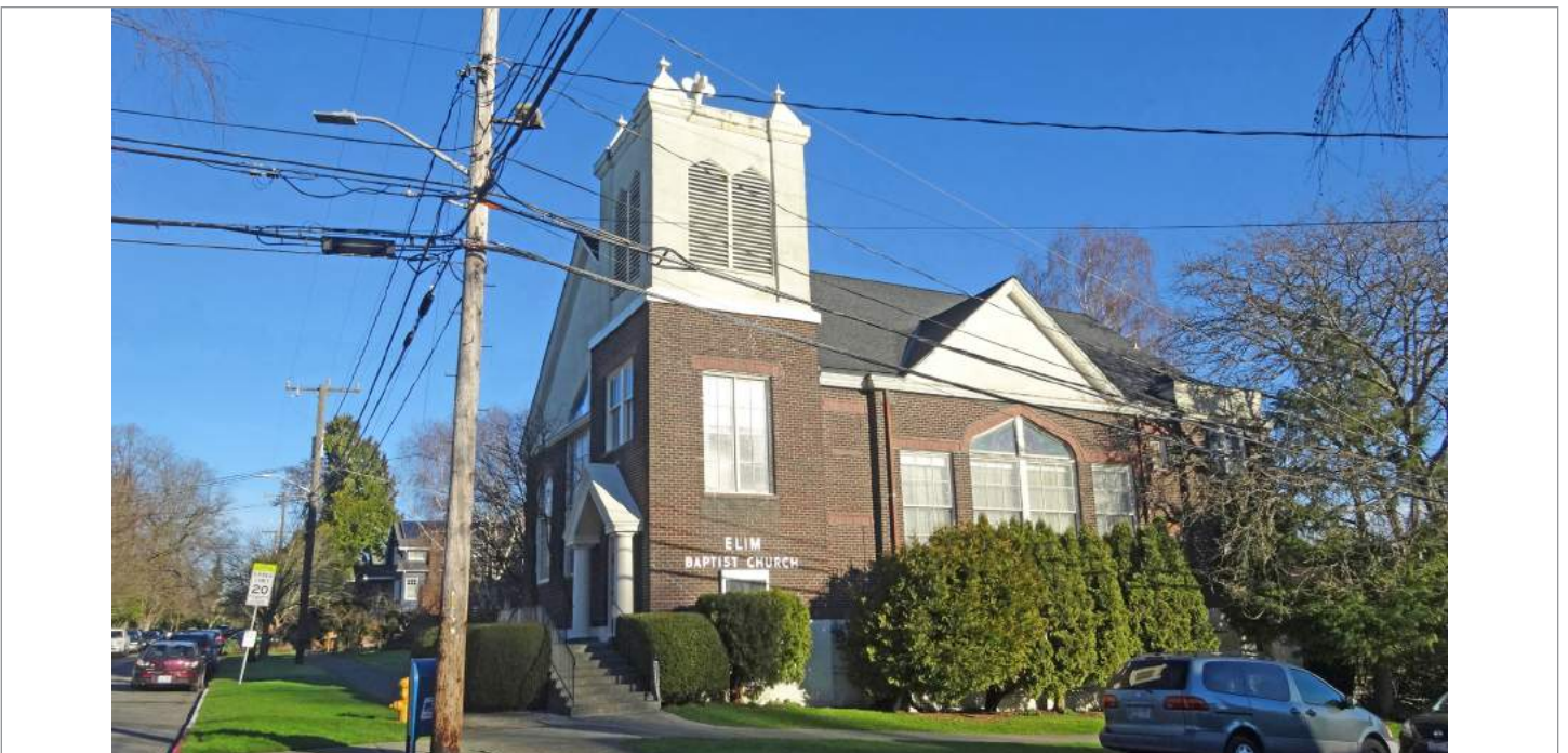
WA_King County_Wallingford-Meridian_Streetcar_HD_0028. Elim Baptist Church, looking north.
