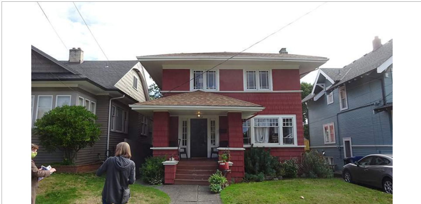
WA_King County_Wallingford-Meridian_Streetcar_HD_0045. 4554 Latona Avenue NE, looking east.
