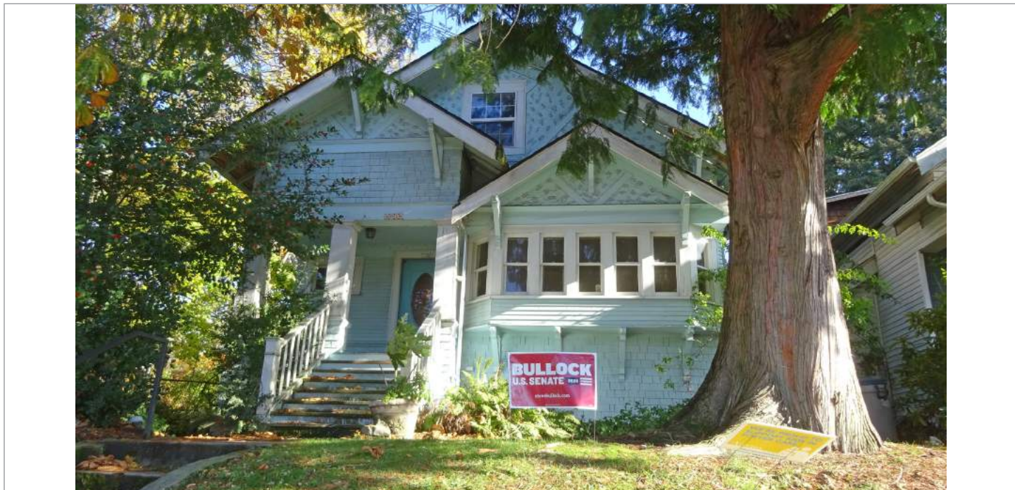
WA_King County_Wallingford-Meridian_Streetcar_HD_0025. 4616 Meridian Avenue N, looking east.
