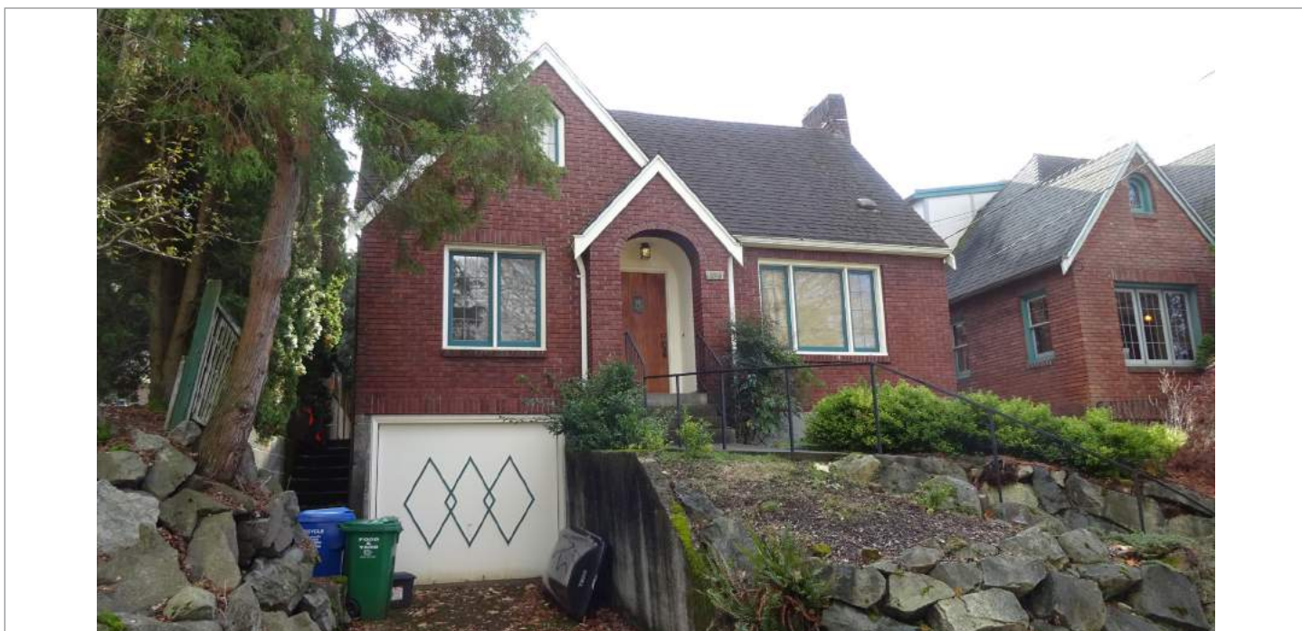
WA_King County_Wallingford-Meridian_Streetcar_HD_0024. 1921 N 48th Avenue, looking southwest.
