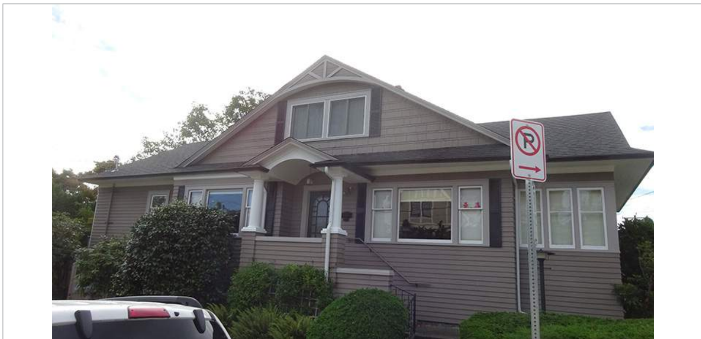
WA_King County_Wallingford-Meridian_Streetcar_HD_0044. 4558 Latona Avenue NE, looking southeast.
