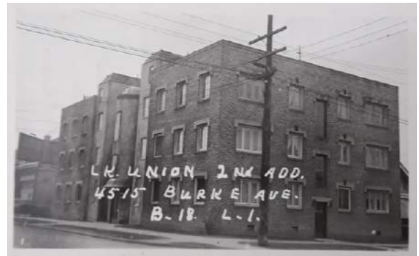
Fig. 15. Multi-family apartment building at 4515 Burke Ave. N, King County Assessor, 1939
