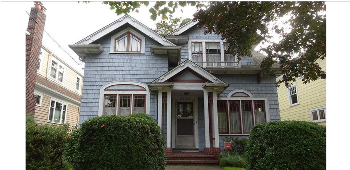
WA_King County_Wallingford-Meridian_Streetcar_HD_0049. 4520 Latona Avenue NE, looking east.
