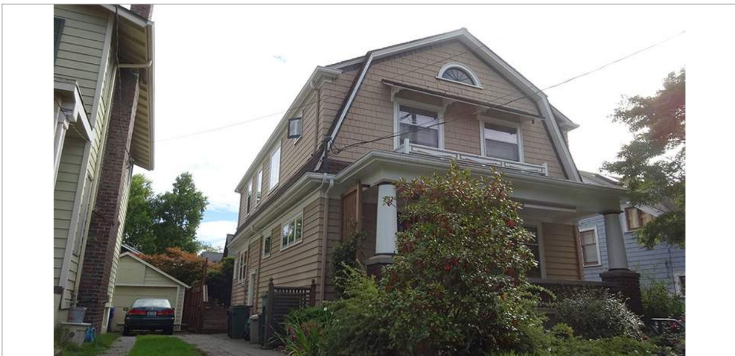
WA_King County_Wallingford-Meridian_Streetcar_HD_0048. 4524 Latona Avenue NE, looking east.
