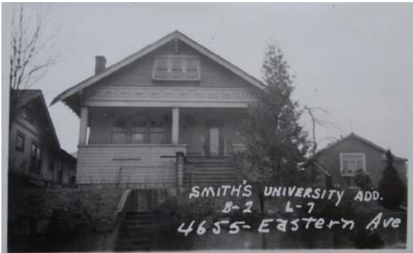
Fig. 8. Craftsman-style residence at 4655 Eastern Ave. N, King County Assessor, 1939
