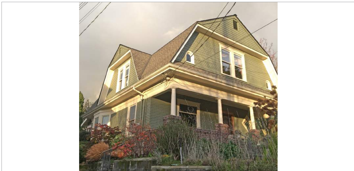
WA_King County_Wallingford-Meridian_Streetcar_HD_0006. 1426 N 47th Street, looking northeast.
