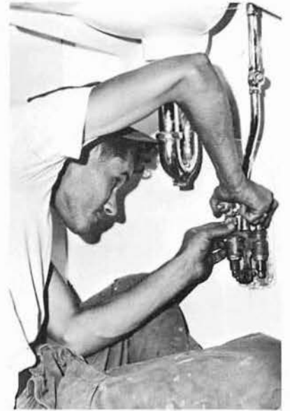
If it leaks, just shut off the water
