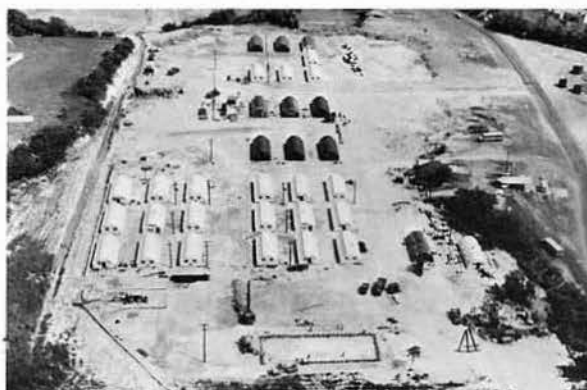
View of project at end of September, 1965
