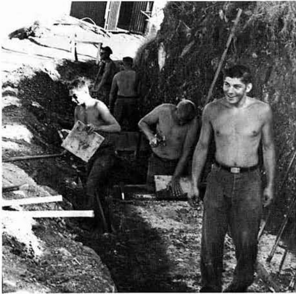
Retaining wall—Crane Hill
