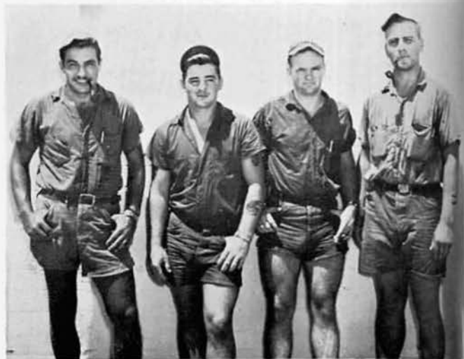
Asphalt tile crew
