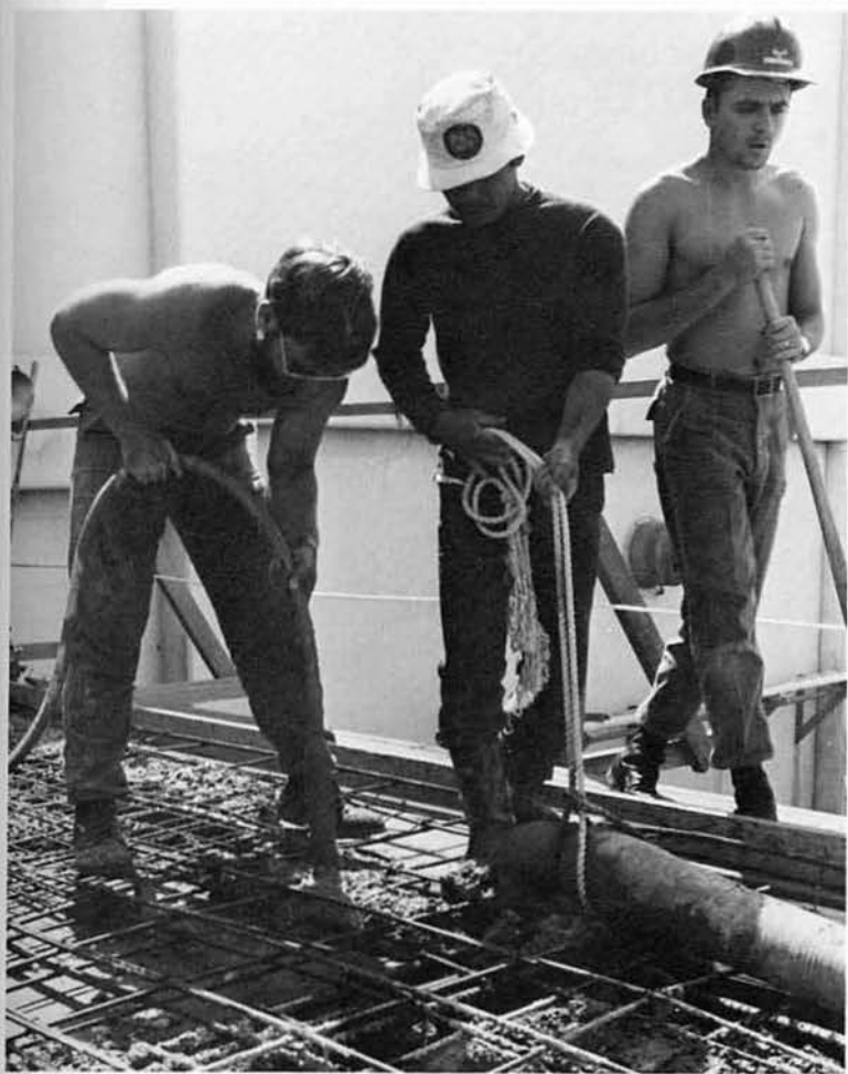
SW3 S. Gilmore (R) and BU2 C. Bazil (L) placed concrete with Japanese National on roof.
