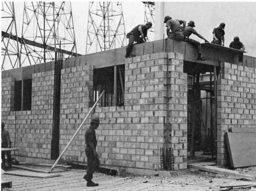
The shop takes shape.
