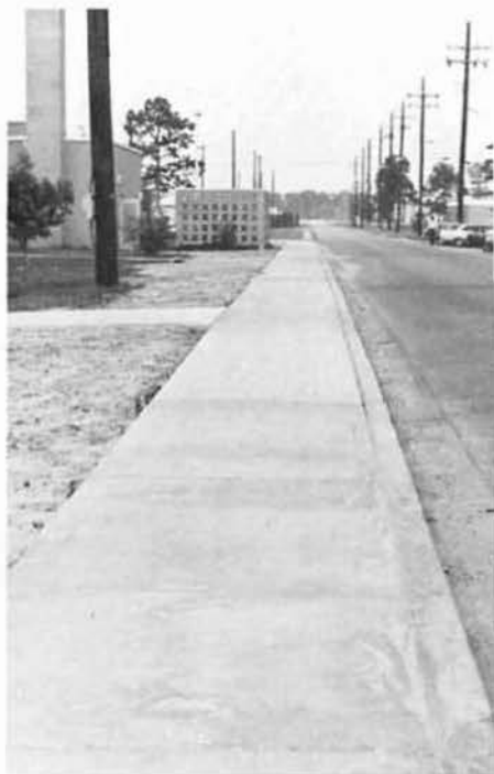
Another "C" Co. Project, 1st street sidewalk.
