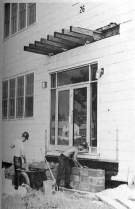
Canopies and Porches were "C" Co.'s gift to the barracks.
