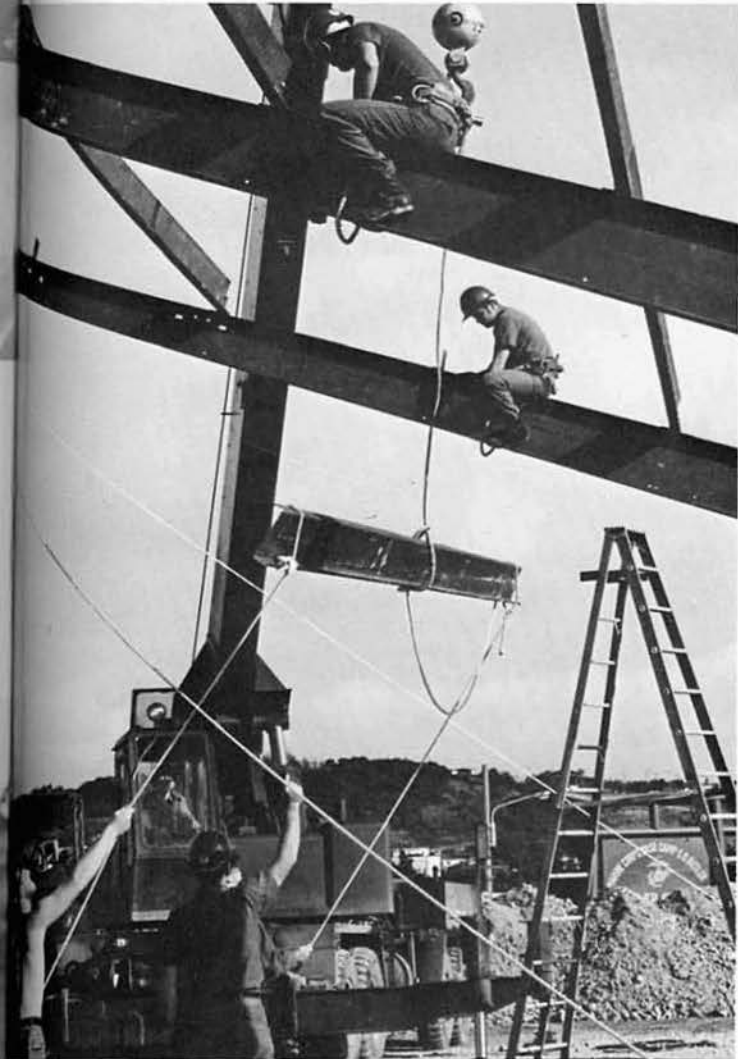
Erecting steel members at Zukeran.
