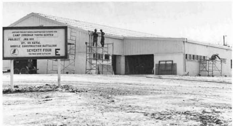
Before we left 86 percent of the project was complete.
