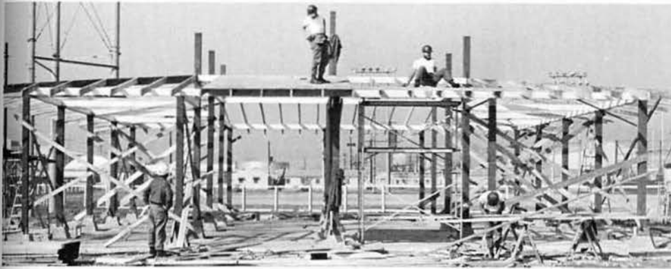
Wingside Picnic Shelter
