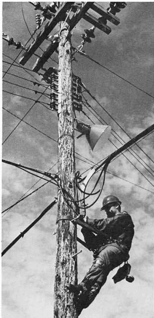
CECN J. Engel of Bravo Co. installing communication lines.
