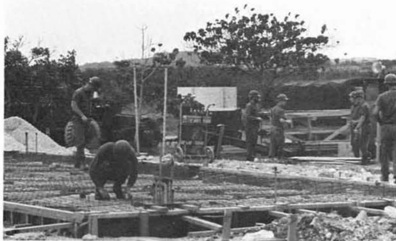
Where's the cement truck?
