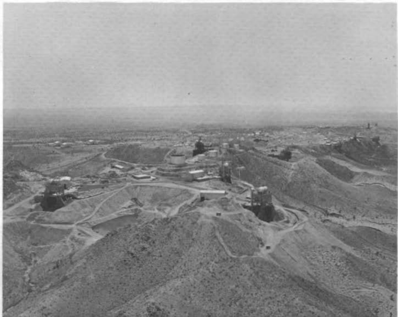
Photo shows new three F-1 test stand addition at NASA High Thrust Area, Edwards California, constructed under supervision of the Los Angeles District, U. S. Army Corps of Engineers. Test Stand 1-E is on left with water recovery reservoir. Also shown is Test Stand 1-D in foreground right and Test Stand 1-C adjacent.
