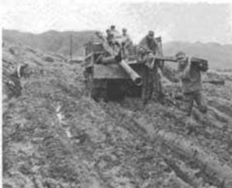
Crew from MCB-FIVE's "Delta" Company installs culverts to improve road conditions.
