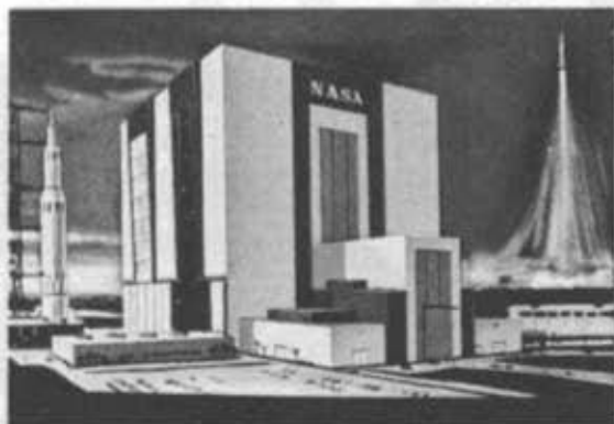
THE VEHICLE ASSEMBLY BUILDING National Aeronautics and Space Administration Merritt Island, Florida
