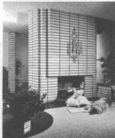
Dutch white Norman brick laid in stack bond with raked joints.
