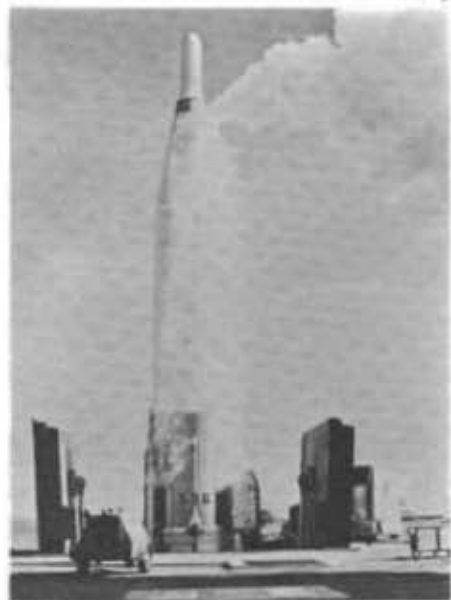
Atlas "F" missile in readiness, over silo built by Utah joint venture.
