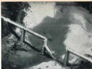
XOM CA TRANG bridge, 60 miles north of the Demilitarized Zone, lost its center span as a result of a direct hit with a Bullpup missile.
