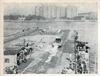
USS INTREPID'S catapults are tested before the ship leaves the New York Naval Shipyard at end of six-month, \$10 million conversion.
