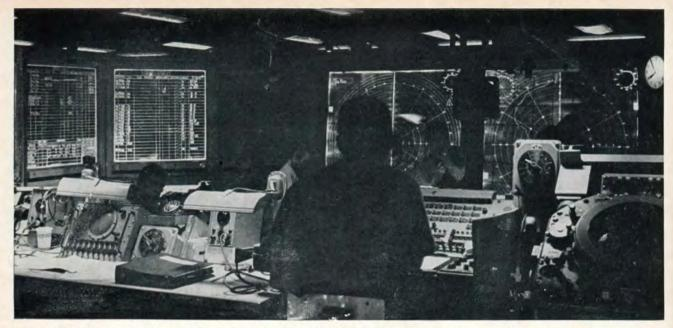
THE COMBAT Information Center, located between the flight deck and the hangar deck in the forward part of the ship, is the hub of
