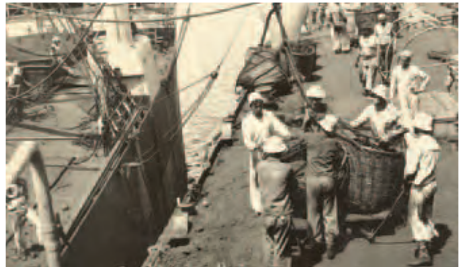
Coaling ship was a dirty job that lasted several days. Derricks lowered bags of coal into bunkers, and Sailors spread out the coal with shovels. It took several days more to clean the coal dust that covered everything and everyone. William Stewart Collection.
