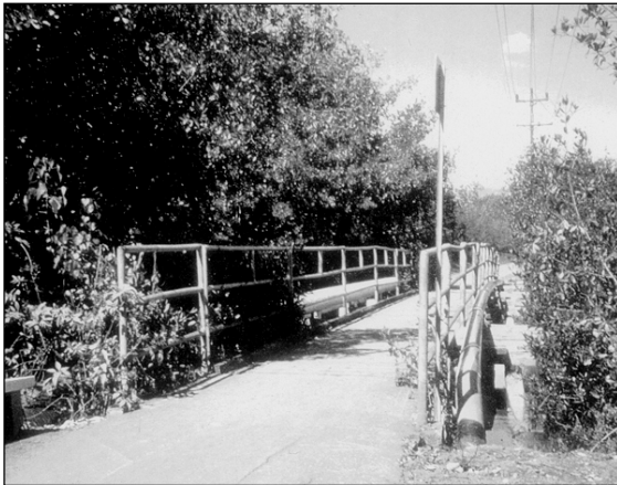
Above and Above Right: The overgrowth of mangrove (above) can be removed to improve safety and to open up shoreline visibility (above right) in some areas along the Trail.
