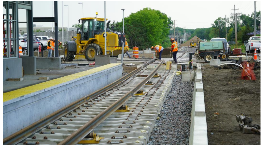
LRT track at the Downtown Hopkins Station
