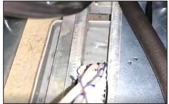
Top View of Drain Piping
