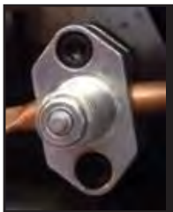
refrigeration line tapping valve
