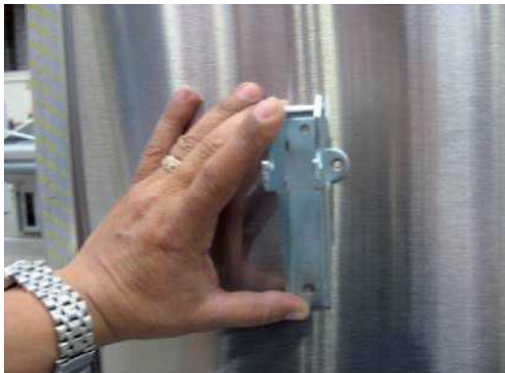
Step 3: Use bracket center hole to align with cross mark.
