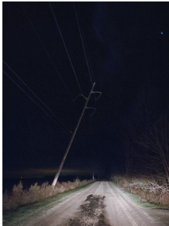
Figure 23: Failed Wood Pole on Circuit S2N
