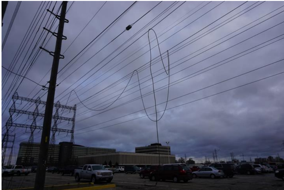
Figure 33: V76R Insulator Failure
