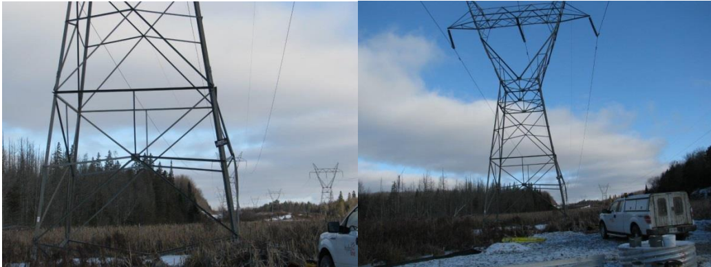
Figure 2: Buckled Legs and Tower Leaning (Circuit M80B, Minden, ON)
