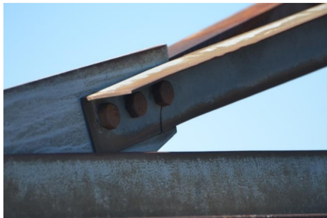
Figure 4: Broken and Cracked hanger examples
