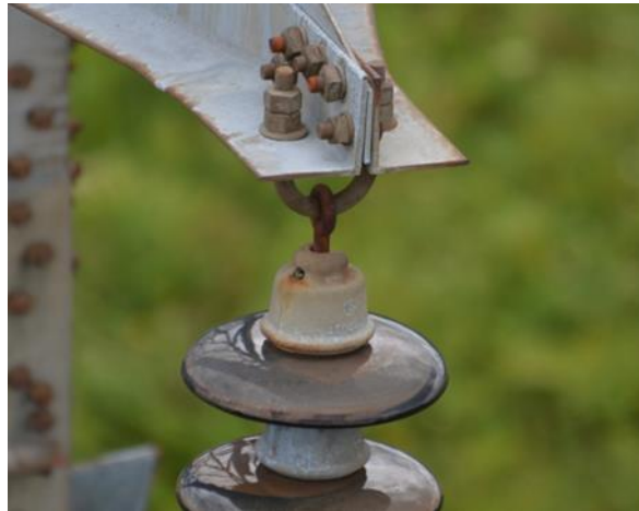
1 Figure 49: U-bolt on a suspension structure
