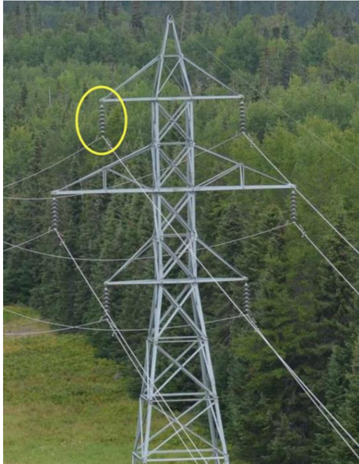
Figure 30: Transmission Line Insulator String
