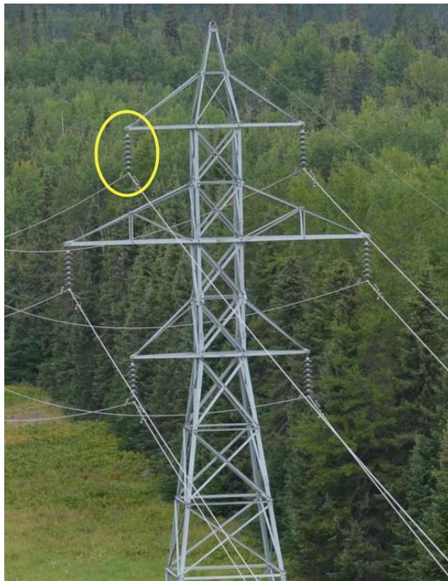
Figure 1: Transmission Line Insulator String
