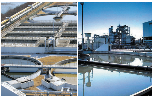
Asan Plant Wastewater Treatment Complex
