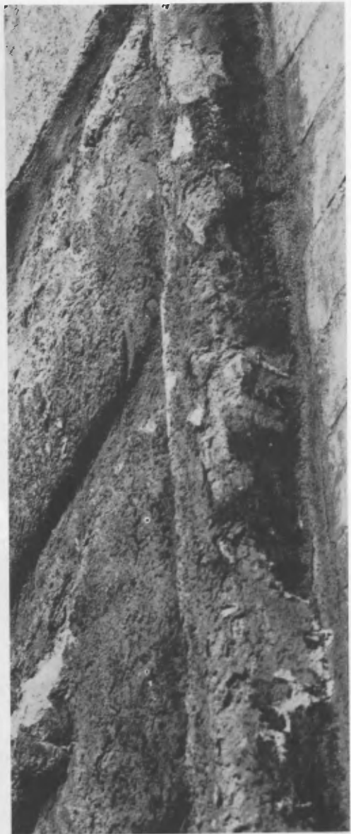
Fig.6 - Palazzo del Podestà, same detail as in Fig.5, today. Note the exfoliated crust still preserved.
