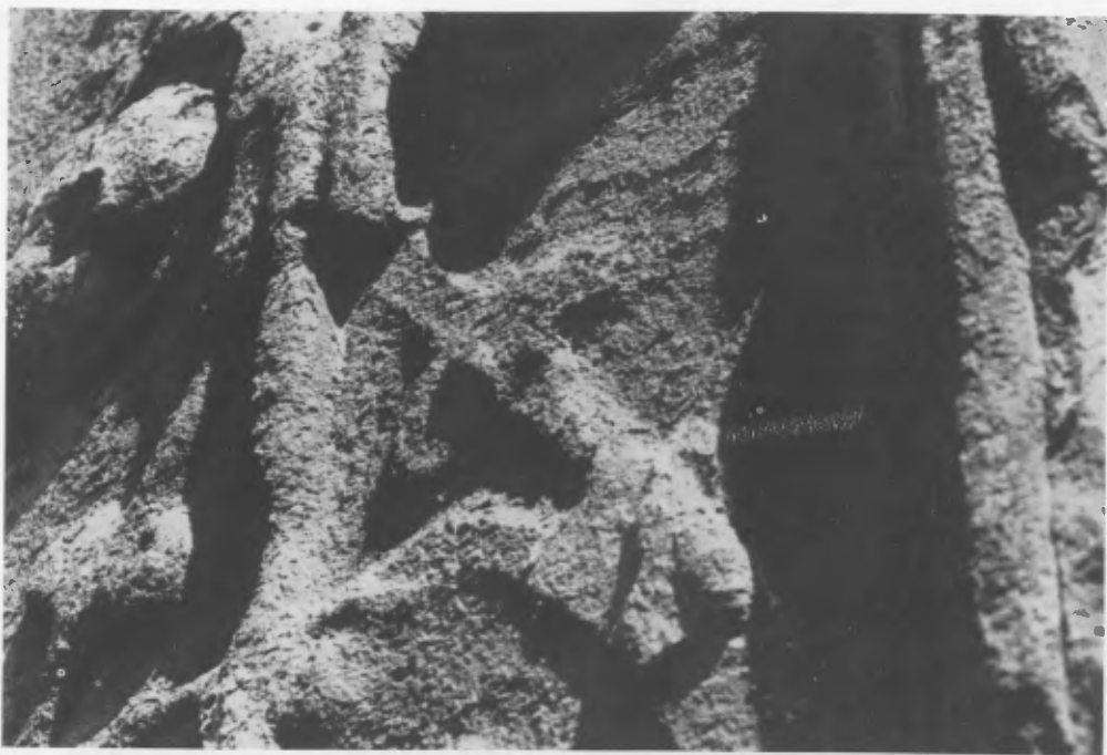
Fig.7 - Palazzo d.Podestà, detail after Rhodorsil treatment.
