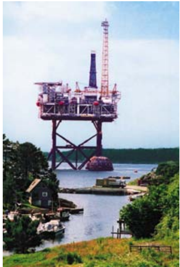
The Maureen production platform, which operated in the United Kingdom sector of the North Sea from 1983 until the field's depletion in 1999, was successfully refloated and towed to Norway for dismantling. The platform, the largest and heaviest nonconcrete structure in the North Sea, was moved safely and without environmental incident.
