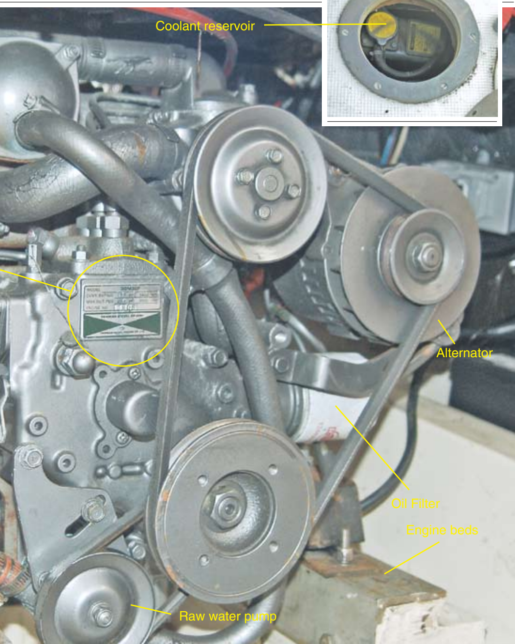
A typical diesel auxiliary (this one's a three-cylinder Yanmar in an old Columbia 36) and some of its various components.
