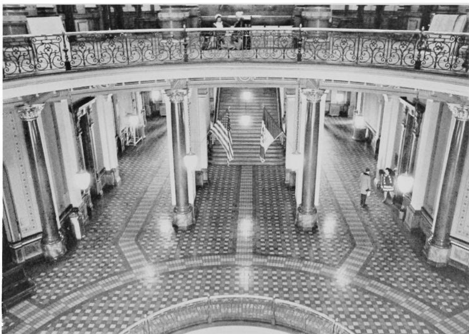
Interior views of Iowa Capitol Building.
