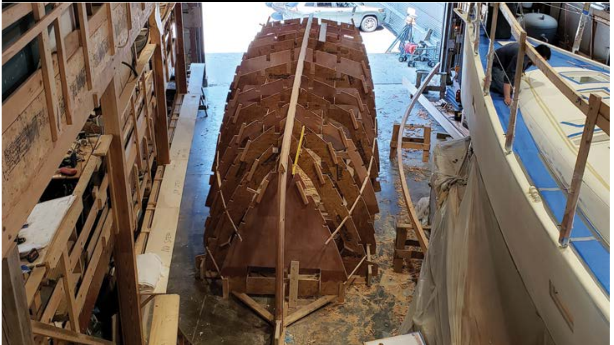
The 38-foot Wheeler under construction at Brooklin Boat Yard in Brooklin. The boat to the right is a new Hinckley Sou'Wester 53.
