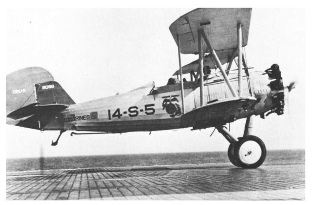
Marine aviation joins the carriers. A Vought O2U-2 of VS-14M on the deck of the USS Saratoga in November 1931. The arresting hook can be seen underneath the fusilage. (Marine Corps Photo 529593).
