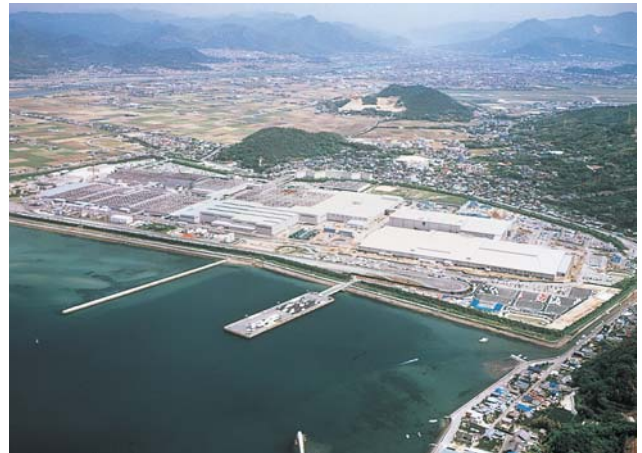
Hofu Plant (Yamaguchi Prefecture)
